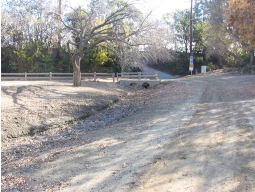
Fig. 3. Dirt culvert in Crystal Springs area (drains to Los Angeles River) which could be restored to a more natural state. Photographed Dec. 2007 by Daniel S. Cooper.
